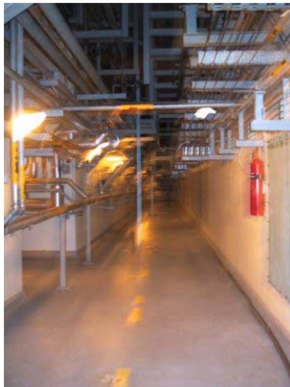
Fig 2 Valve Maintenance Access Area – Corridor EA51
